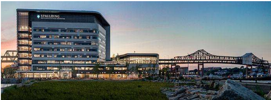
Figura 26. Spaulding Rehabilitation Hospital. Fonte: Health Facilities Magazine
